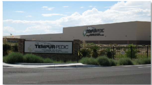
Tempur-Pedic Manufacturing Plant
